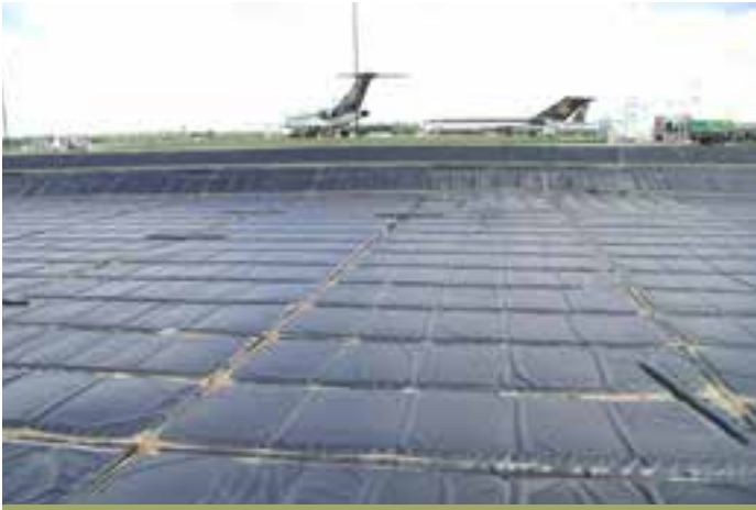
Permeable floating cover at sewage
