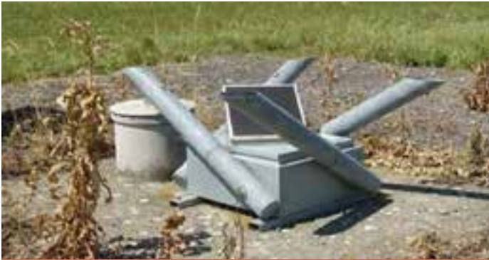
An underground stationary gas powered noise generator
