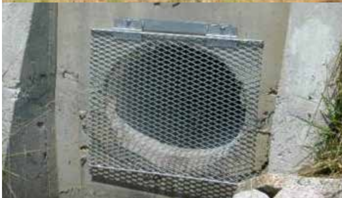
Floating balls and bird netting to cover the water, and drainage opening protection
