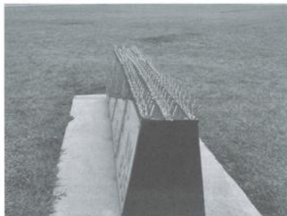
Fig. 4.3. Perching deterrents often include sharpened spikes affixed to areas attractive to birds; shown here is one such deterrent atop an airport sign. Photo credit: Todd Stewart
