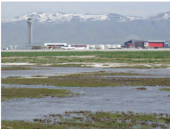
FIGURE 25 Standing water and cattail growth along edge of airfield drainage ditch (Source: BASH Inc.).
