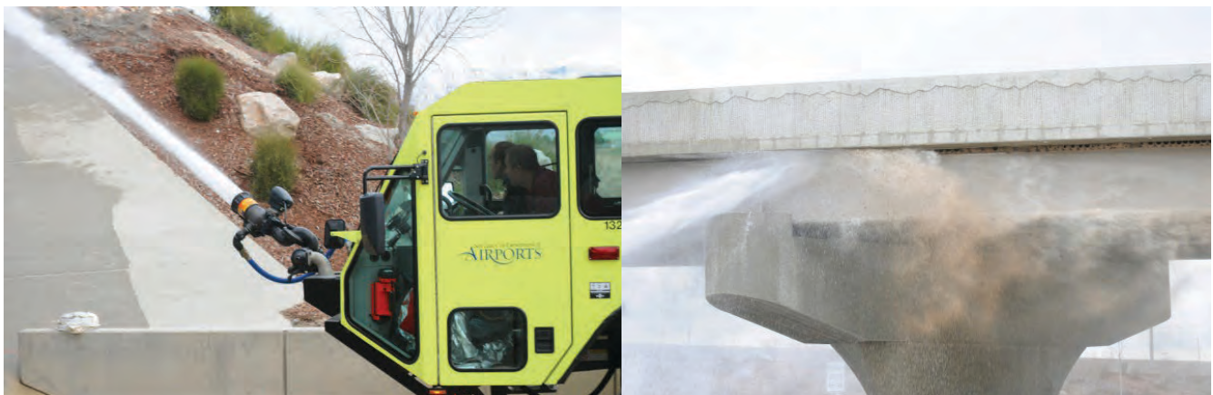
FIGURE 19 Water cannon use to remove cliff swallow nests under support structures at SLC (Source: SLC).
