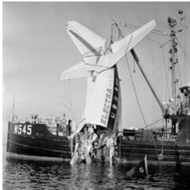
Wreckage of Eastern Airlines Flight 375 as a result of a bird strike with European Starlings, Boston, MA, 4 October 1960
